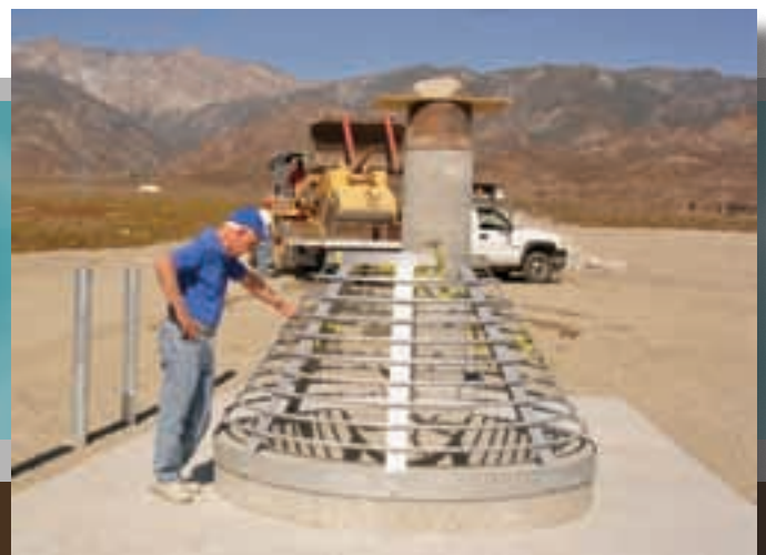
Construction of air gap at Etiwanda Debris Basin.
