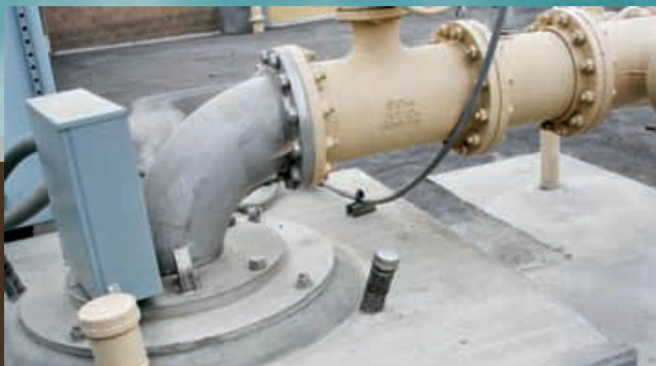
Desalter II sounding tube to be used for transducer installation.
