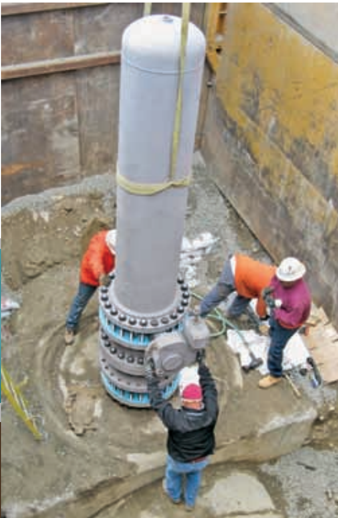
Installation of MWD CB-14 connection.
